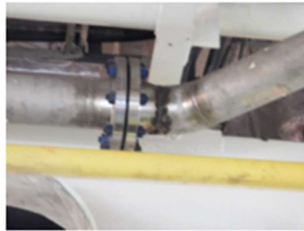
Initial condition of pipework
