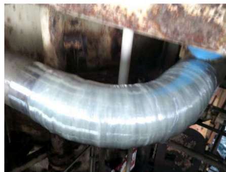
During repair application
