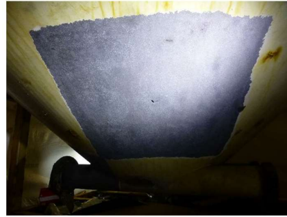
Initial status of tank body – Patch 1
