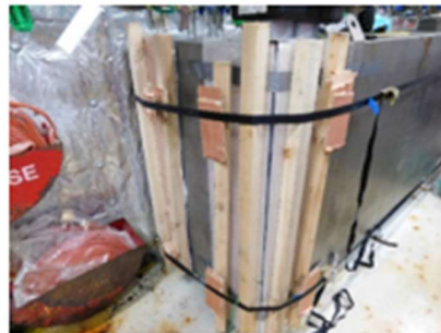
During repair application
