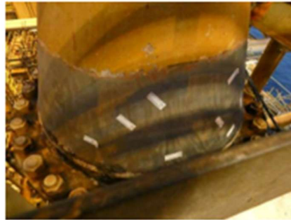
After surface preparation
