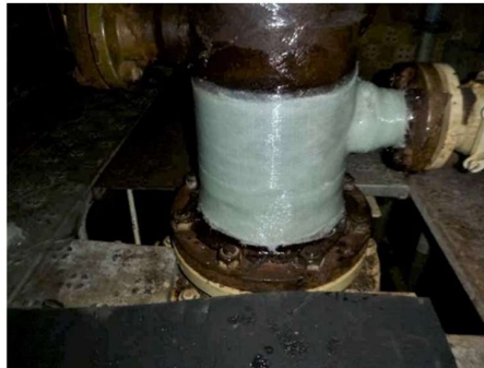
During repair application
