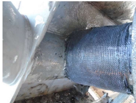
During repair application
