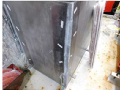
After surface preparation
