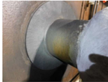
After surface preparation and profiling
