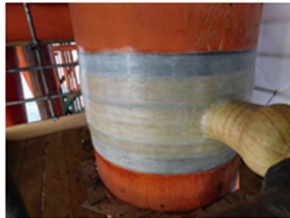
During repair installation
