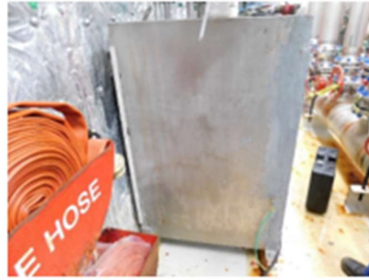
Initial status of tank
