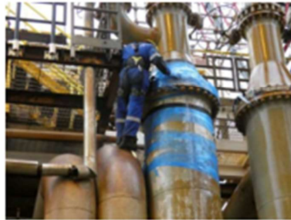
During repair application
