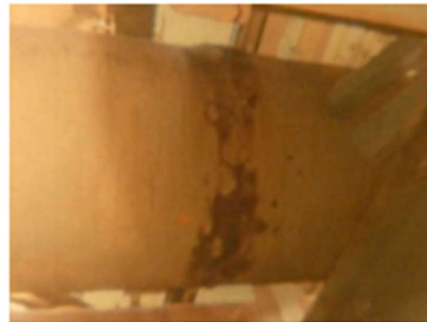
Initial condition of pipework
