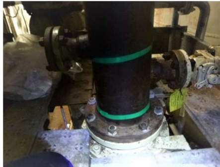
Initial condition of pipework
