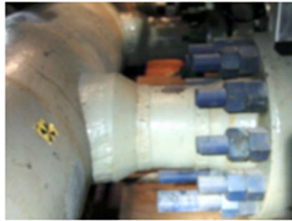
Original status of pipework
