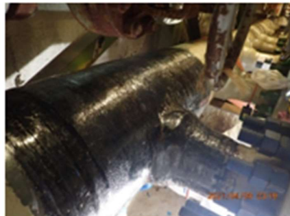
During repair application
