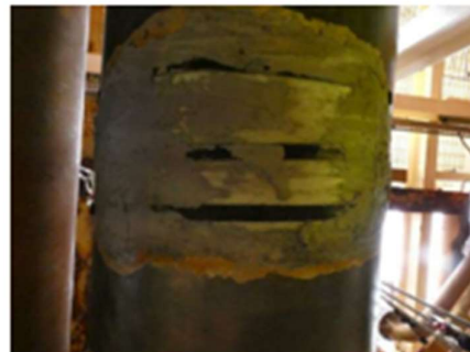
During repair application
