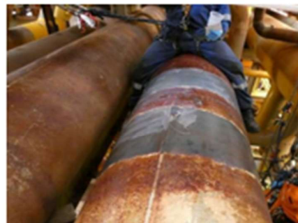
After surface preparation
