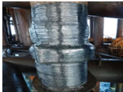
Final cured repair
