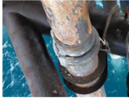
Initial condition of pipework
