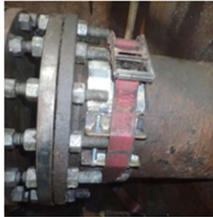
Initial condition of pipework with sealing clamp
