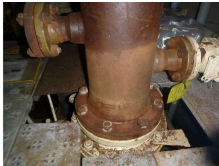
After surface preparation
