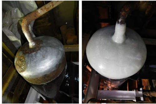
Repair 1 - Initial condition, final repair
