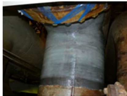
During repair application
