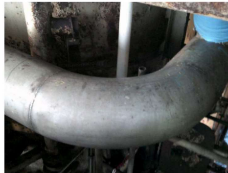
Initial condition of pipework
