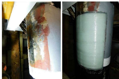
Repair 3 - Initial condition, final repair
