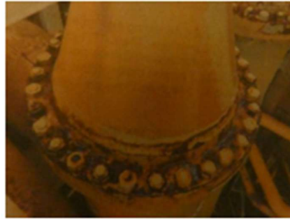
Initial condition of pipework
