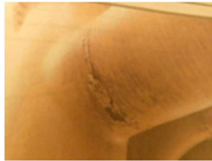
Initial condition of pipework
