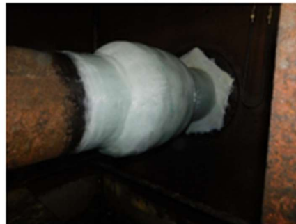
Final cured repair
