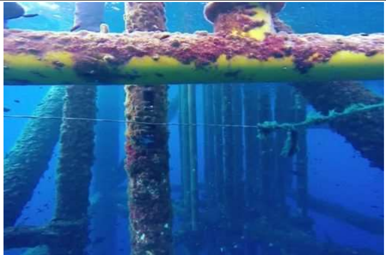
Subsea - Repairing structural components, pipework, pipelines caissons risers.
