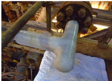
During repair application
