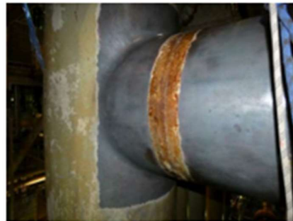
After surface preparation
