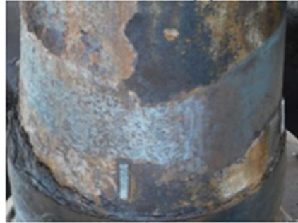
After surface preparation
