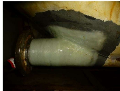
Completed repair – tank pipework
