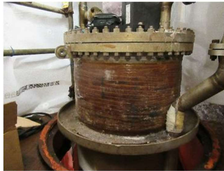
Initial condition of pipework
