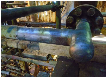
After surface preparation
