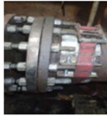
Initial condition of pipework
