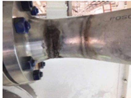
After surface preparation
