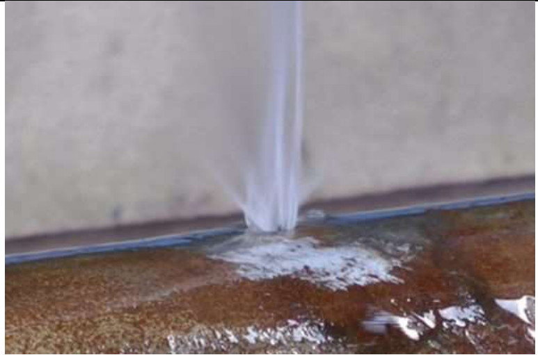
Live Leak Sealing - Repairs topside or subsea components with live leaks.
