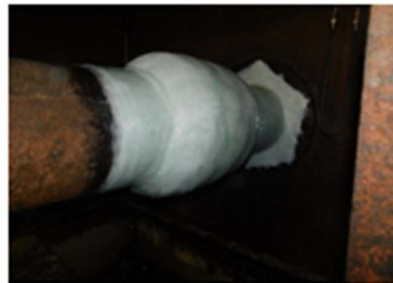
During repair application
