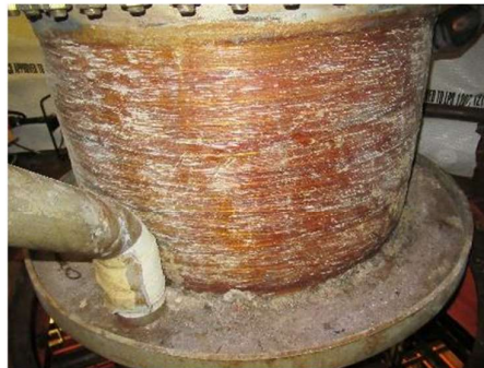
After surface preparation
