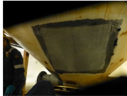
Completed repair – Patch 1
