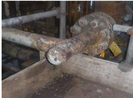
Initial condition of pipework
