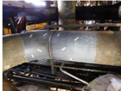
Initial condition of pipework
