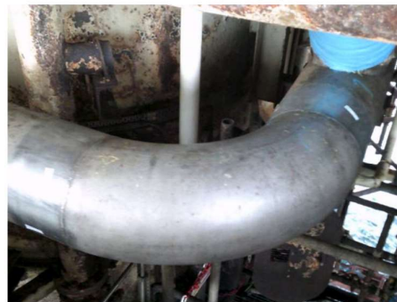
After surface preparation
