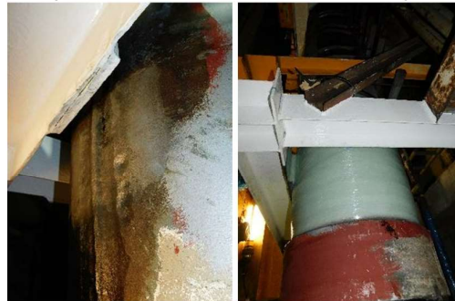
Repair 2 - Initial condition, final repair
