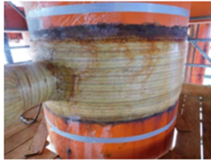
Initial condition of pipework and repair
