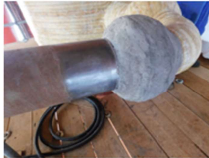
After surface preparation and profiling
