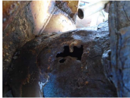
Initial condition of stub
