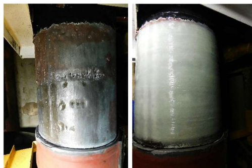
Repair 4 - Initial condition, final repair
