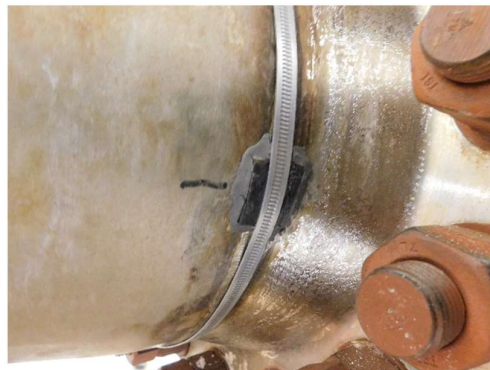
After surface preparation and profiling
