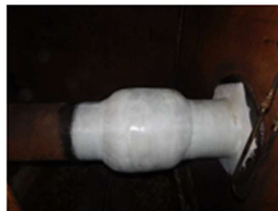
Final cured repair
